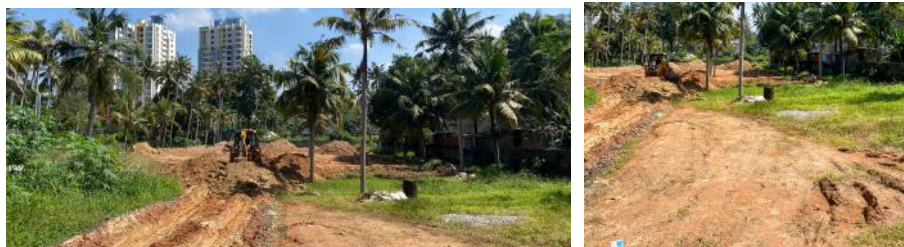
Plot development in progress by Dhan L4 lands at Attinkuzhi, Kazhakkootam
